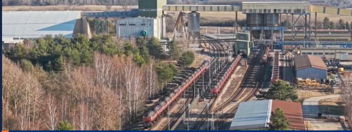
Rail loading yard at the smelter
